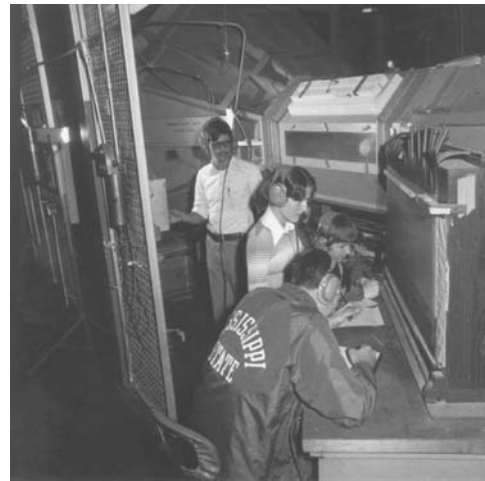
Fig. 9 Students working in the subsonic wind tunnel in the 1970s
